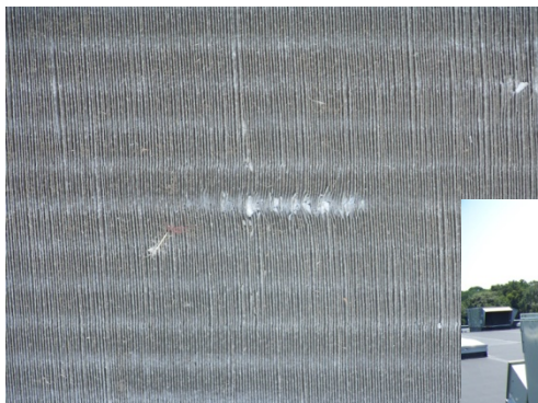
Above: Ocean facing MicroGuard coated condensing fins after 7 years
