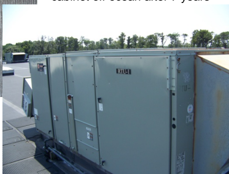
Below: MicroGuard coated cabinet off ocean after 7 years
